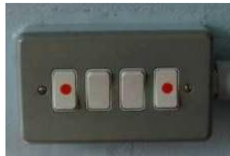
Light switches labelled up with red dots – 'never switch on'
